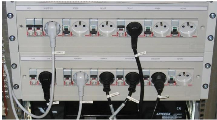
Example of the labeling of a power box with circuit breakers and power sockets.
